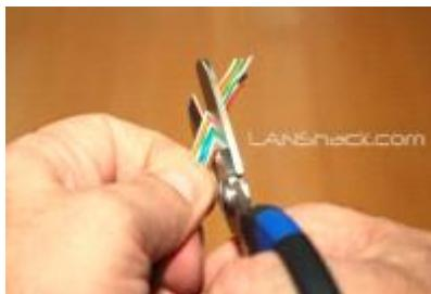
7. **TEC-TIP:** Cut the wires on a very sharp angle to make it easier to install the load-bar(in the next step).
